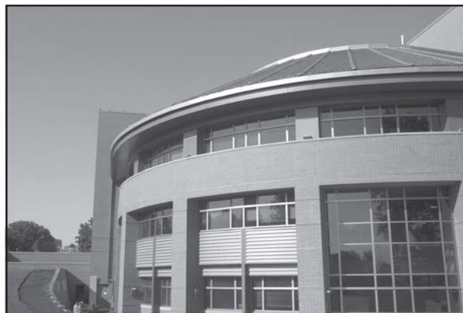
Addition to the McCollum Science Building.
